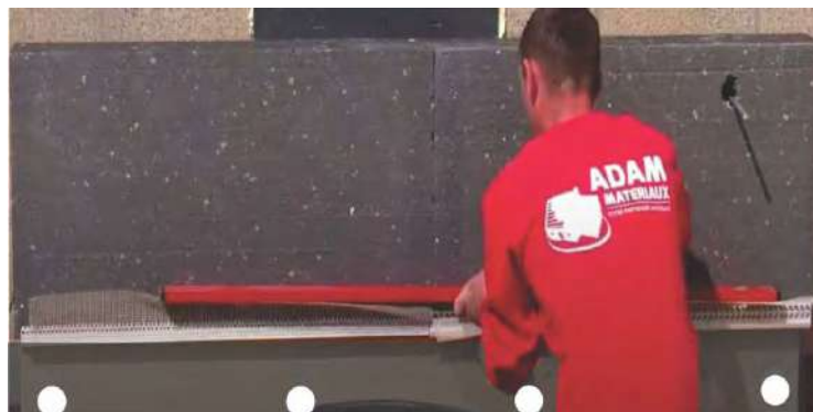
Installation of EPS 032 Adam Materiaux insulation - EPS HD Adam Materiaux
