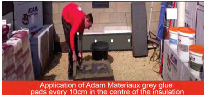
Application of Adam Materiaux gray glue for bonding EPS Adam Materiaux
