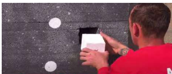
Passage of the electric cable through the EPS block Adam Matériaux
