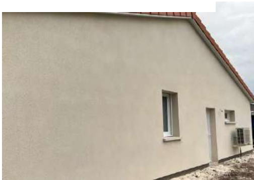
Well-placed roof overhang
