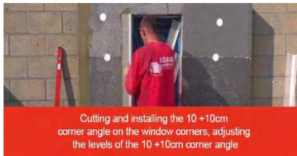
Same technique for installing the LK PVC Premium 10x10cm facade corner bracket around windows and doors.
