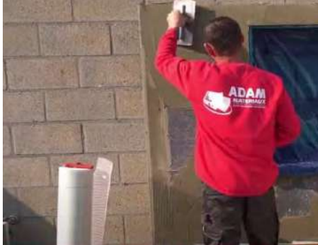
Using Kubala 0202 6x6mm plaster
