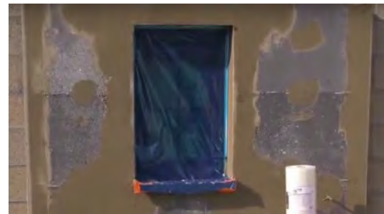
Same technique for installing the LK PVC Premium 10x10cm facade corner bracket around windows and doors.
