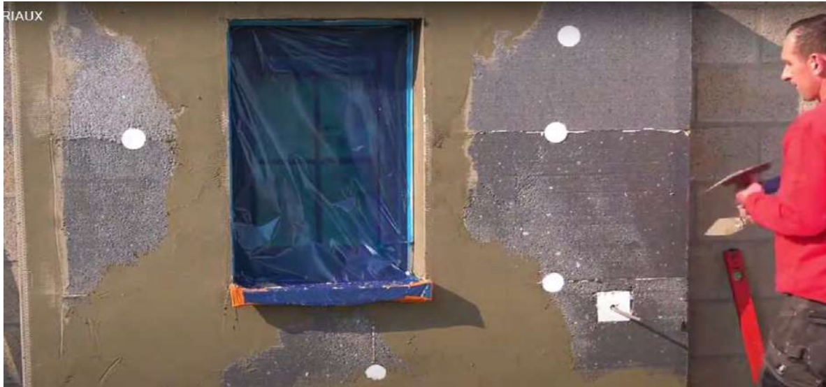
EPS plugs placed in the Adam Matériaux EPS insulation BEFORE the installation of “bandages” using Adam Matériaux gray or white glue .
