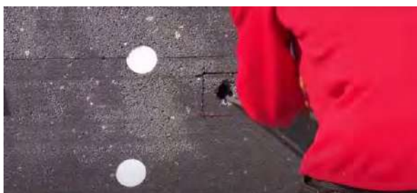
Installation of a custom-made block for fixing the lamp, alarm, attachment, ...
