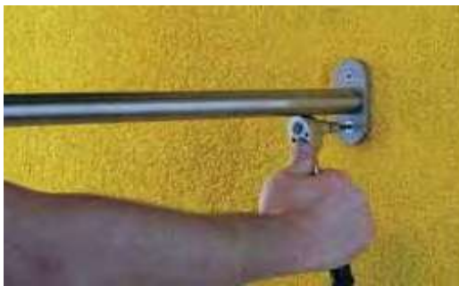
Installation of railings fixed to the UMP blocks after laying the plaster
