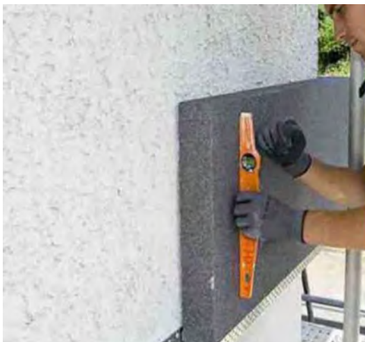
Using a level for laying Adam Matériaux EPS
