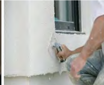
Applying plaster with Kubala 0300
