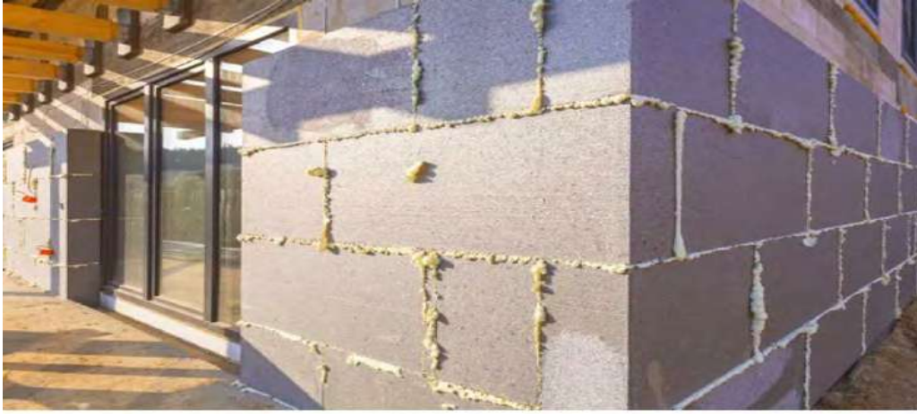
Installation of Adam Matériaux EPS insulation in a staggered pattern, in the correct manner
