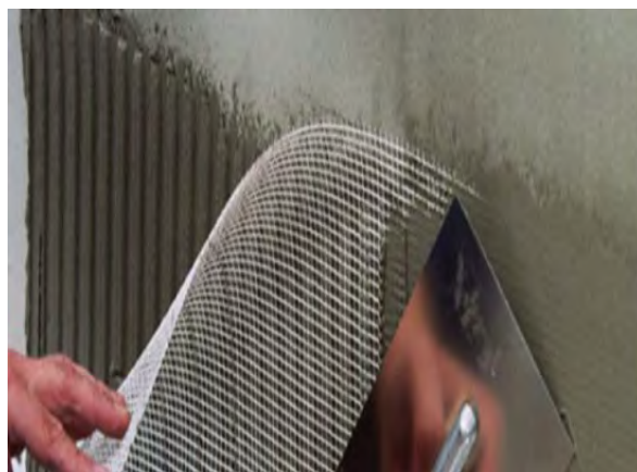
Crushing the Adam Materiaux reinforcement net into the Adam Materiaux gray or white glue
