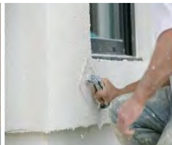
Applying plaster with Kubala 0300
