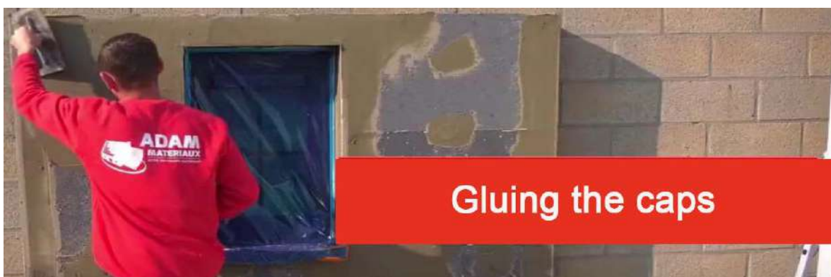
Applying "bandages" using Adam Matériaux gray or white glue to close the EPS caps placed to "drown" the fixing dowels.
