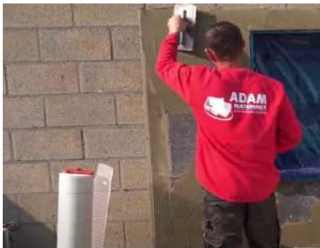
Using Kubala 0202 6x6mm plaster
