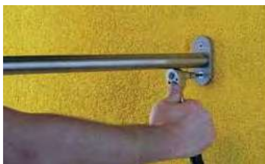
Installation of railings fixed to the UMP blocks after laying the plaster
