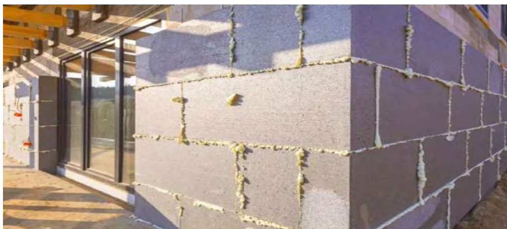
Installation of Adam Matériaux EPS insulation in a staggered pattern, in the correct manner
